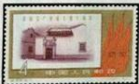
Congress Building, Shanghai — A151
