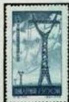
High-tension Pylon — A53
