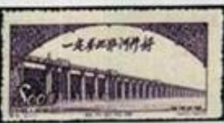
Huai River Sluice Dam A29
