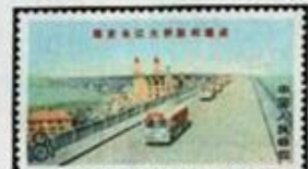
Road across Bridge — A252
